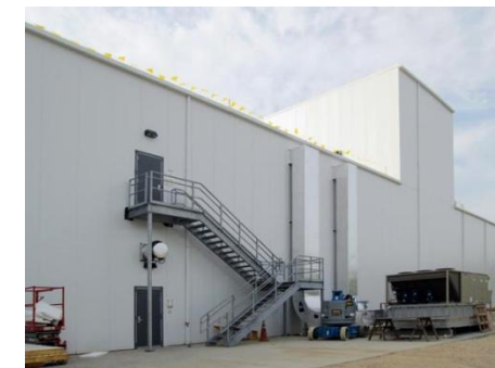
Peptide Plant in USA
