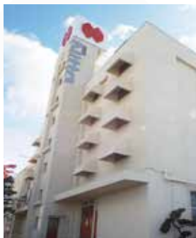
Head Office and Osaka Plant
