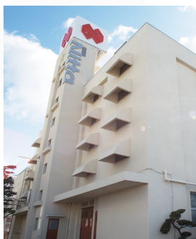
Head Office and Osaka Plant
